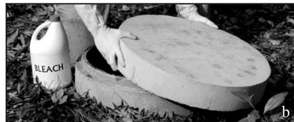
**3.** Take the containers of bleach and funnel (if needed) and carefully pour all the bleach down into the well casing.
