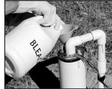
**4.** After the bleach has been added, run water from an outside hose into the well casing until you smell chlorine coming from the hose. Then turn off the outside hose.
